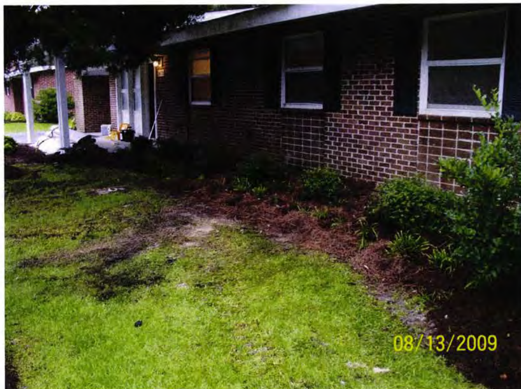
Picture 2: UST 1473Cardinal site after completion of work.
