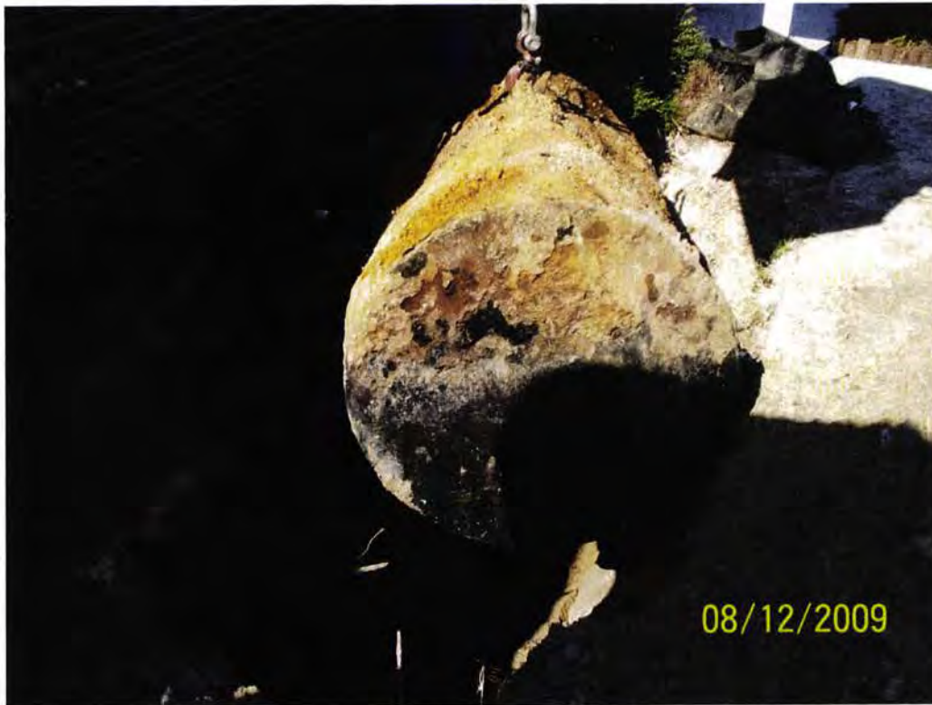
Picture 1: UST 1473Cardinal tank during excavation.
